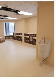
Infection Control Handwash Sinks have been installed between stations. Shown is a pair of dialysis stations, west end.
