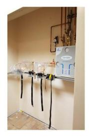
Oxygen Cylinder room near the receiving dock. Bottled Oxygen is piped to the unit at all stations
