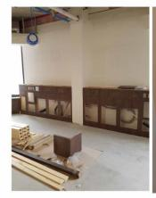
Millwork being installed at all patient treatment stations. The millwork serves as a chase for plumbing and electrical work.
