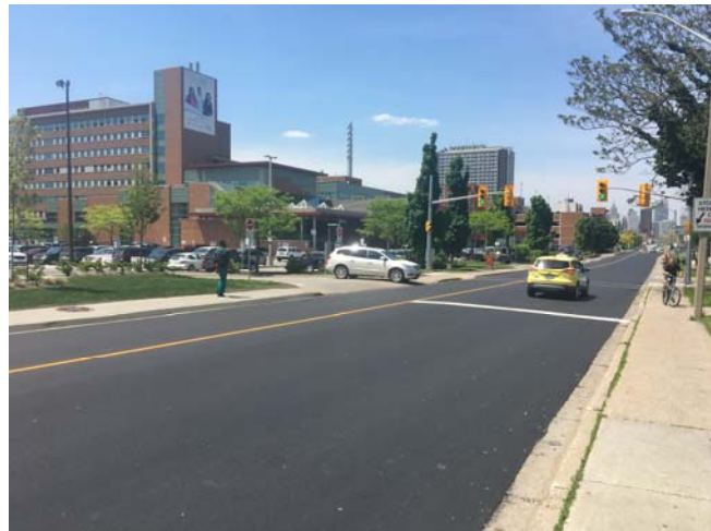
Photo above: View looking down Goyeau Street with newly paved road.
