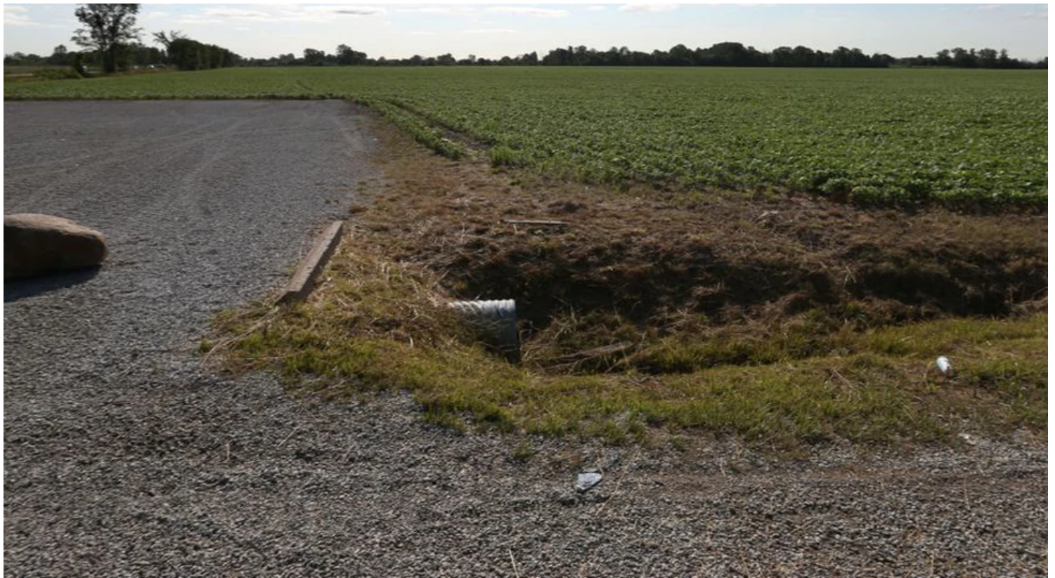
Site of the new mega-hospital to be built on County Rd. 42 at 9th Concession in Windsor, Ont. (JASON KRYK/The Windsor Star)
