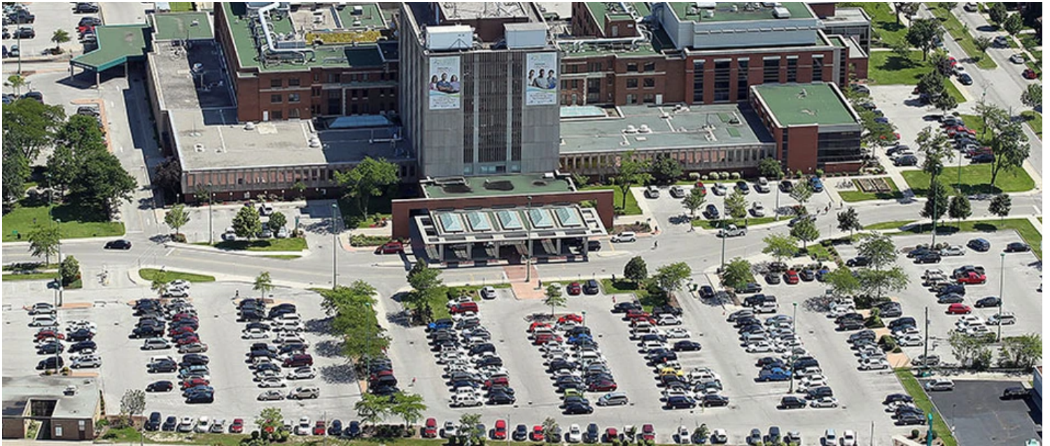
The Windsor Regional Hospital MET campus is seen in Windsor on Wednesday, July 15, 2015. (TYLER BROWNBRIDGE/The Windsor Star)
