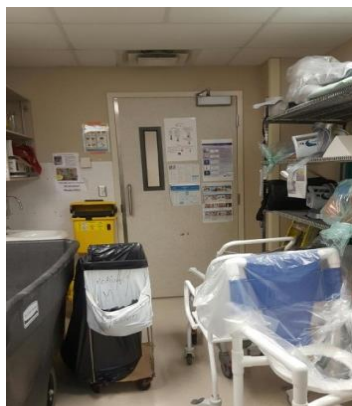
Soiled Utility Supply Room – 8E, Ouellette
