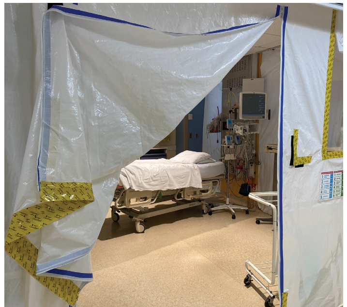
Improved control over ventilation systems and more isolation rooms eliminates the need for so-called “tented rooms,” which WRH installed to improve ventilation during the pandemic.
